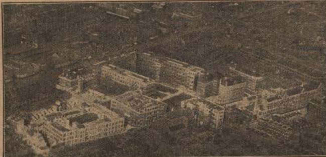
THE BIGGEST HOSPITAL IN ENGLAND.
